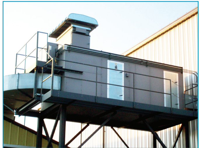
Heating-Only Application for Weld Smoke Removal
