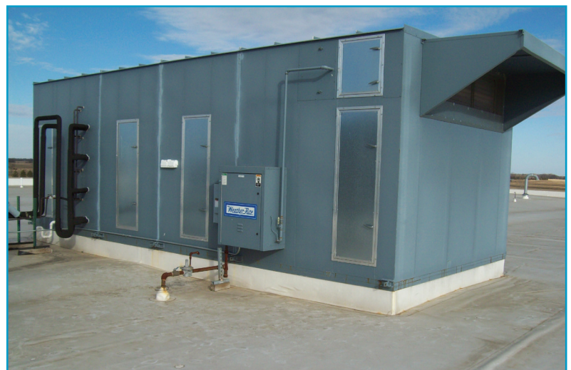
Customized Unit for Heating, Cooling and Make-Up Air
